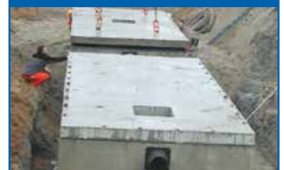
Terreinafwatering asfalt Rotterdam
